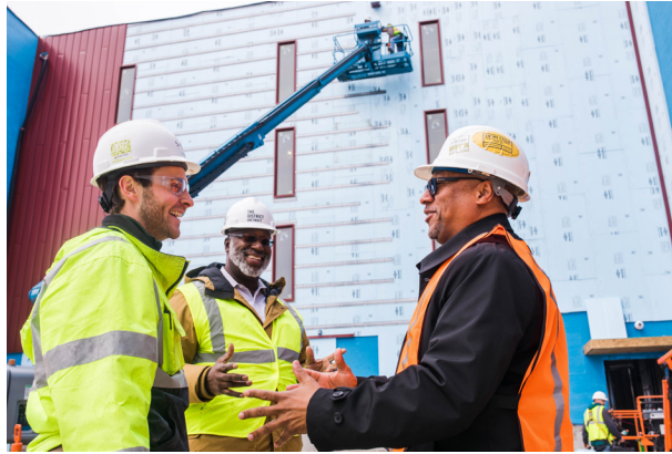
Construction images show progress
